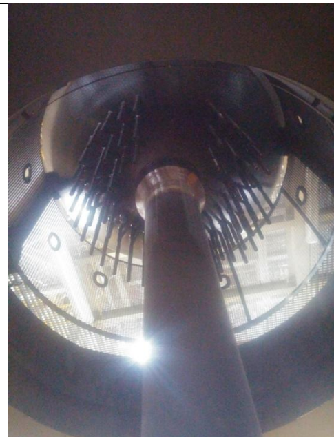
FIGURE 9: BOTTOM OF THE PRESSURISER
